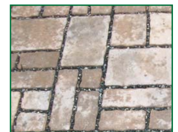
Permeable Pavers contribute to responsible water management by lessening the impact of storm water run off as well as increasing on site infiltration.
