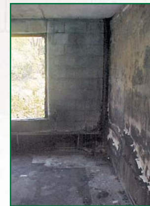
Compartmentation with concrete masonry for multi-residential structures provides protection by preventing the spread of fire from one unit to the next. This conserves life, property and valuable natural resources.
