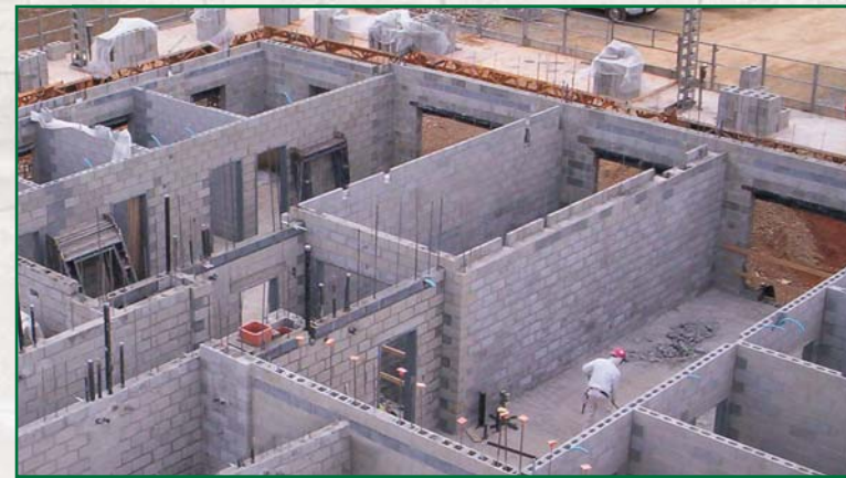
Compartmentation with concrete masonry for multi-residential structures provides protection by preventing the spread of fire from one unit to the next. This conserves life, property and valuable natural resources.
